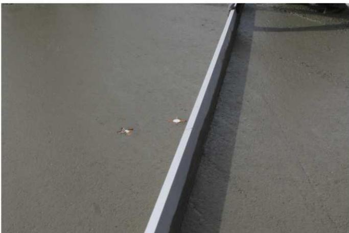
1. Check the location of the measurement point and the required measurement depths from the installation plan.
